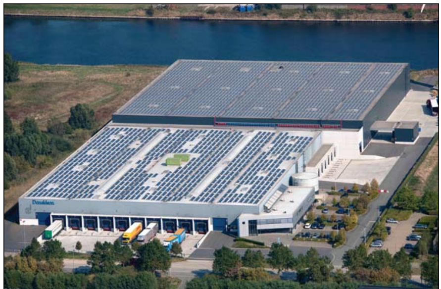
An Enfinity solar rooftop installation producing 803 MWp per year.
