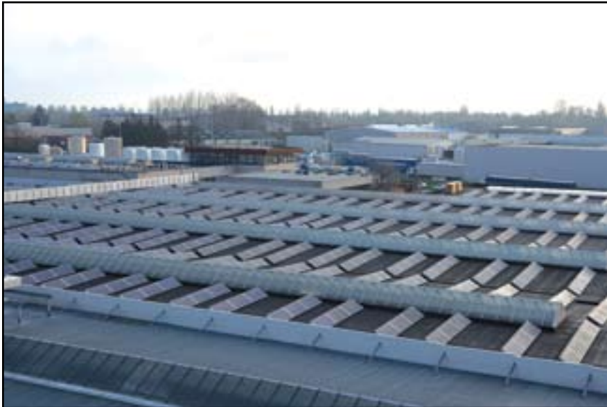
This manufacturing facility has 1.2 MWp of solar energy on its rooftop.
