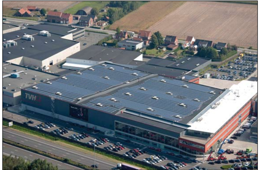
A 604 kWp solar rooftop installation by Enfinity.
